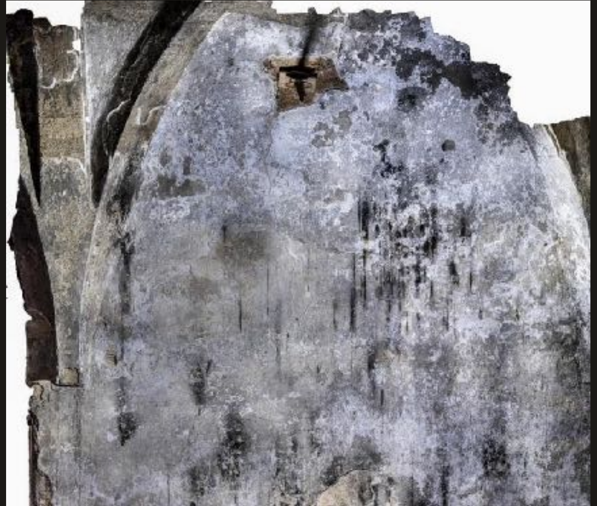
South wall, section S1: wall-surface model
